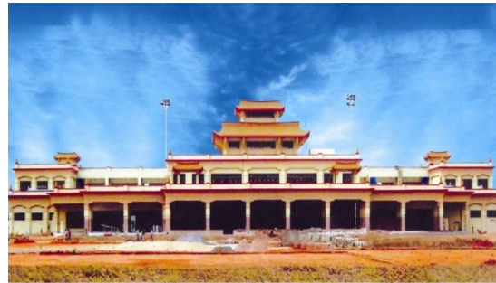
NEW TERMINAL BUILDING AT GAYA AIRPORT, GAYA
