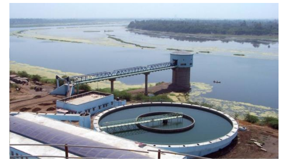
WSS AT VARIAV - VIEW OF 10M DIA INTAKE WELL IN 15M DEEP RIVERBED WITH 14M DIA PUMPHOUSE & 60MLD WTP
